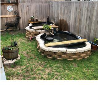
is about 18" tall. I used two of the large ponds from Home Depot that I ordered. I used garden wall bricks to build walls and then capped them with the white stones. I have one pump in the bottom pond
